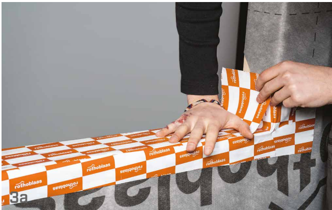
Seal the window with rothoblaas flashing tape.
