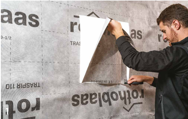
Cut out windows openings.
