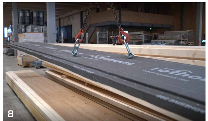
8 The panels prepared in this way are easily transported to the construction site.
