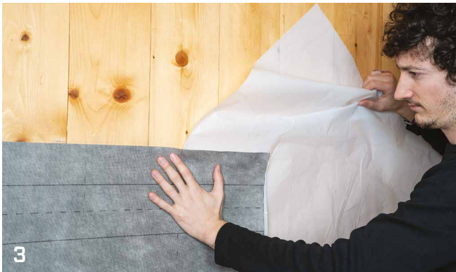
3 Remove release liner and adhere to the substrate from top down.
