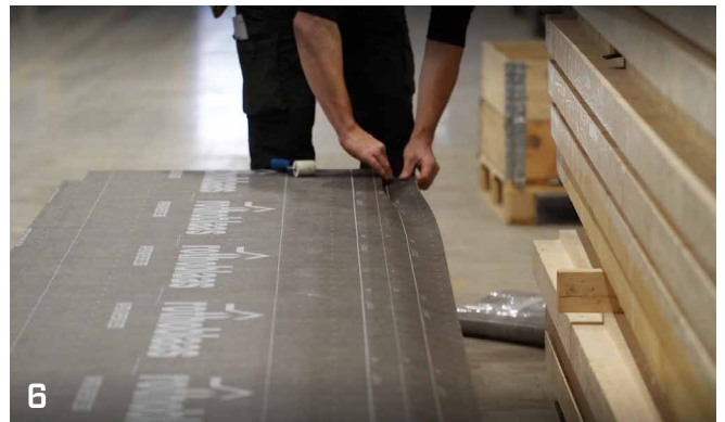
6 Adhesive membrane must wrap the entire panel.
