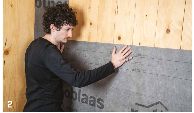
2 Unroll the membrane and apply it on the panel. Use roller to improve the adhesion on substrate.
