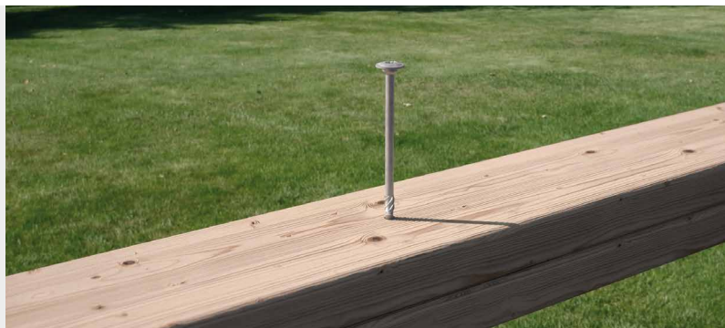
Fastening Wood Trusses outdoors.
