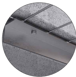
steel angle bracket 30 x 30 x 3 mm
