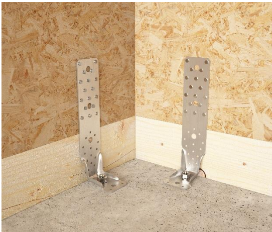
Figure B. 32 Typical installation WKR285
