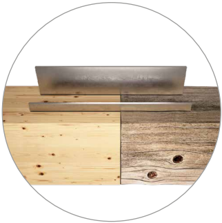
4. REHABILITATION OF DAMAGED PARTS
