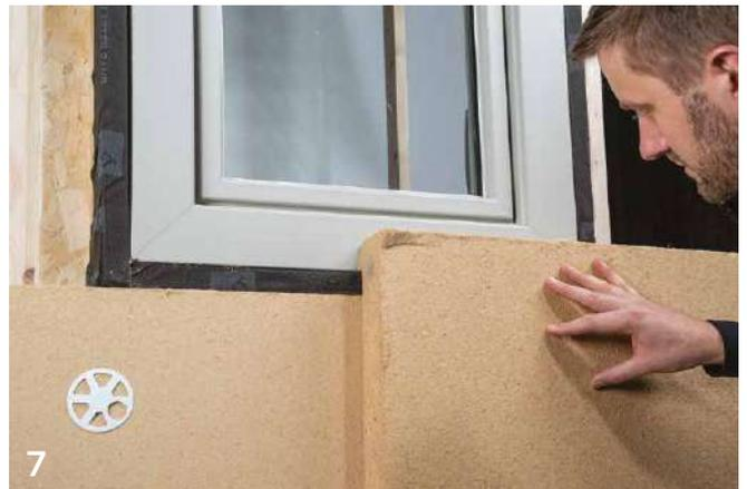
4 EXPAND BAND, WINDOW BAND, FRAME BAND
